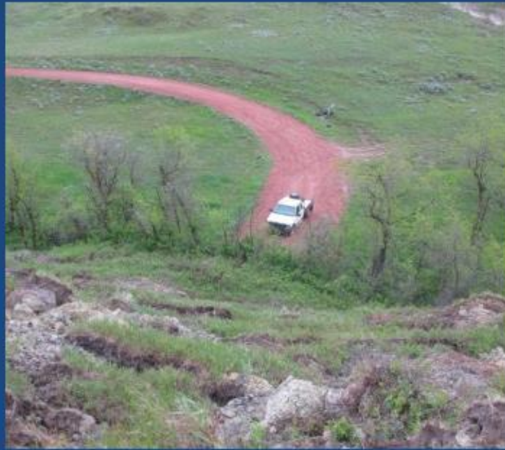
Landslide blocks road winding up to the top of Sentinel Butte, blocking access to a dozen steel towers which provide an important communication link for cellphones and State Radio dispatch (Bismarck Tribune, 2011).
