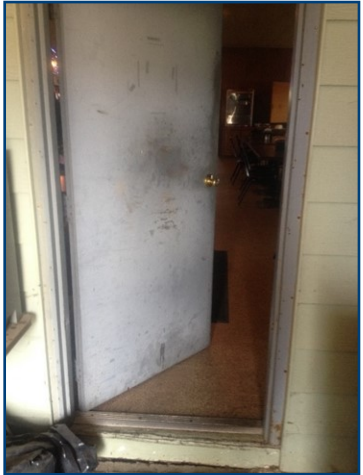
This photo shows an inward swinging door with an incorrect door knob, step down at the door, and a mat that could cause the door from not opening.
