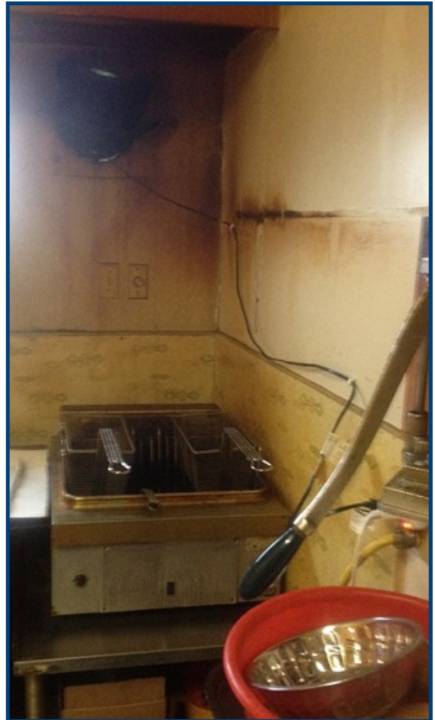
This kitchen photo shows multiple problems -- no exhaust hood or automatic fire protection system in the hood system; a small fan with a very small cord running across the hot vapor space; materials too close to the fryer; a hot fryer next to a wall; an overloaded circuit; and poorly placed switches.
