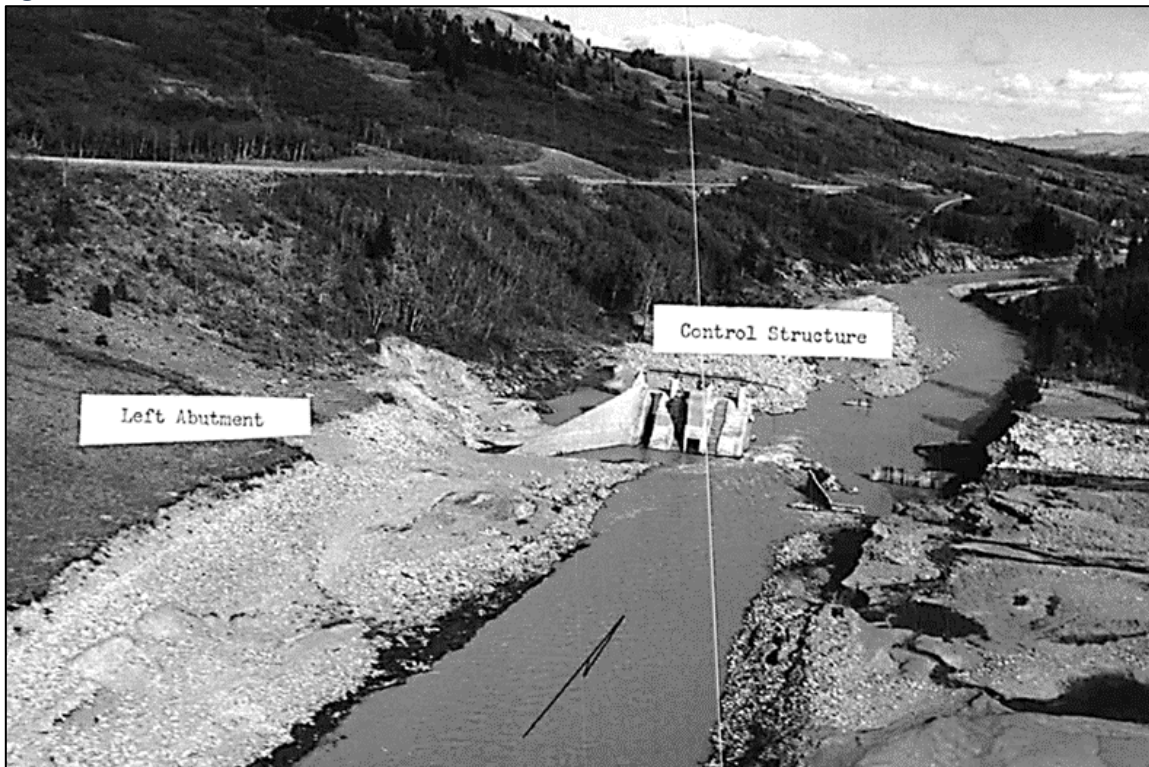
Figure 4.8-15: Two Medicine Dam after failure, Montana, 1964
