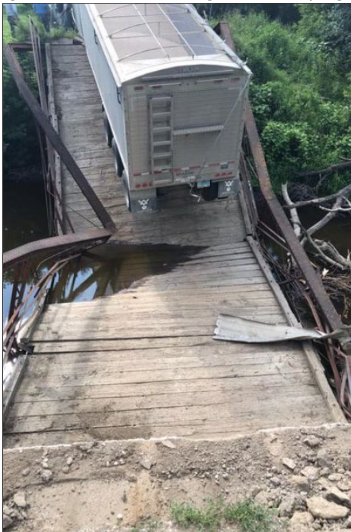
Figure 4.15-4: Northwood historic bridge fails under heavy weight.
