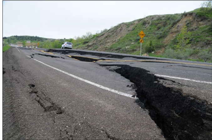
Figure 4.12-9: Highway 22 slumping, near Killdeer
