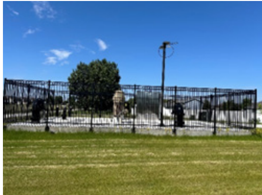
Metro's Lift Station 55 and 56 Project FM-22-C1
